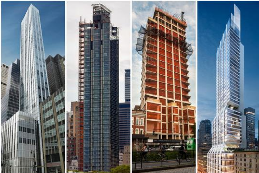
From left: A rendering of 610 Lexington Avenue, a condominium at 53rd Street; 50 United Nations Plaza, a 43-story condominium; 551 West 21st Street under construction; and a rendering of 425 Park Avenue, a 47-story office building at 55th Street.
